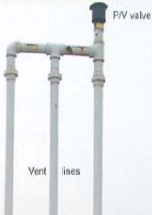
Three vent lines manifolded into one.
